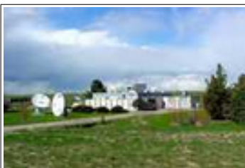
The WWV Building near Fort Collins, Colorado. [Photo courtesy of NIST]
