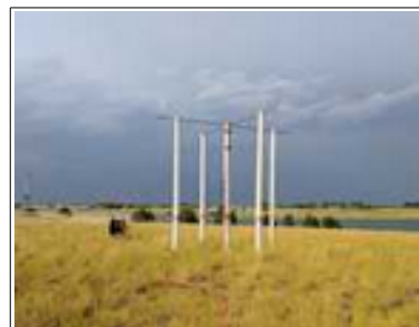
The WWV 25 MHz turnstile antenna. [Matt Deutch, N0RGT, photo]
