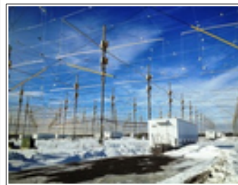
Part of the massive antenna field at the HAARP facility near Gakona, Alaska. The row of white structures contains individual transmitters.
